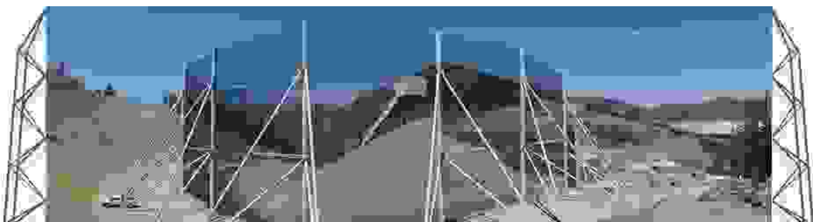
Figure 6.2: Windscreen for dust control (Sharma, 2013)
